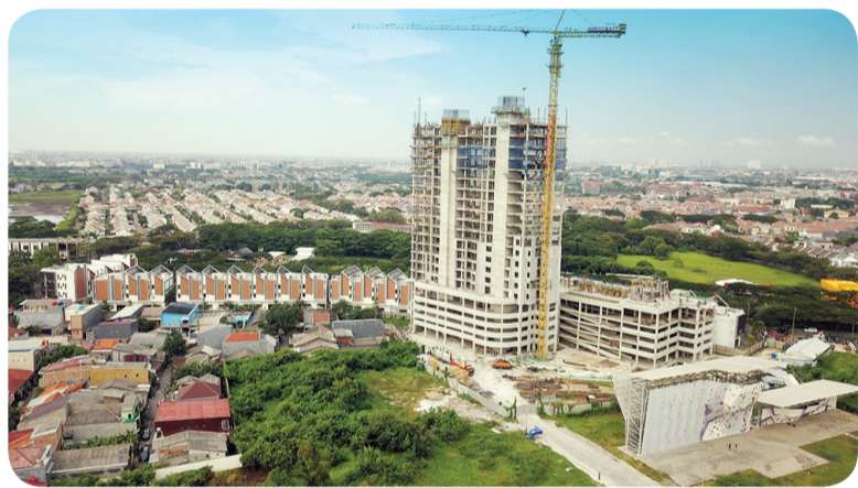
Progress Cleon Park Apartment.
